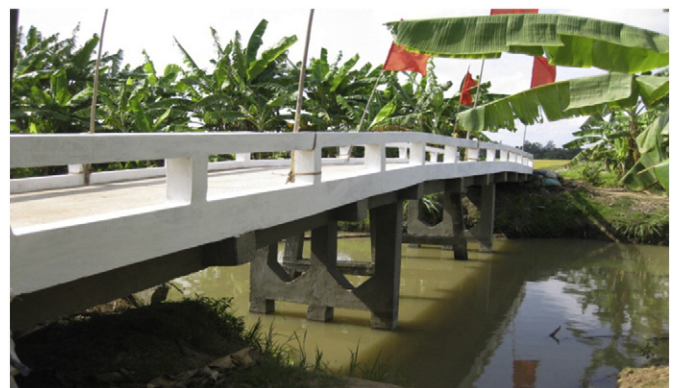
Fig. 3. The concrete bridge built from the 2009's contribution.
